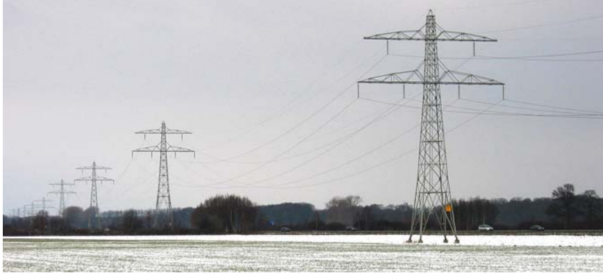
Figure 1. Overhead transmission lines. Spans are suspended between towers from suspension strings.
